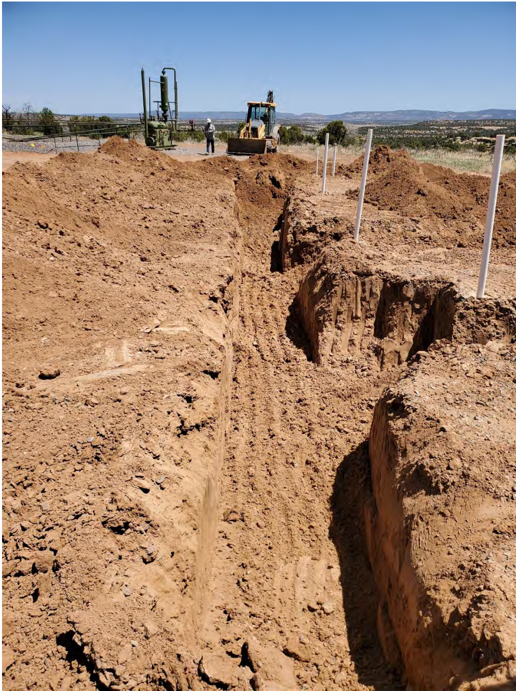
Photo 1: Trenching for piping lay down.
