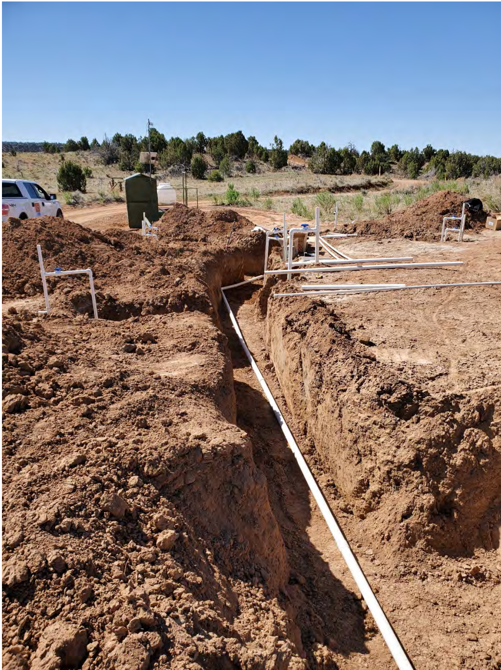
Photo 2: SVE piping install.
