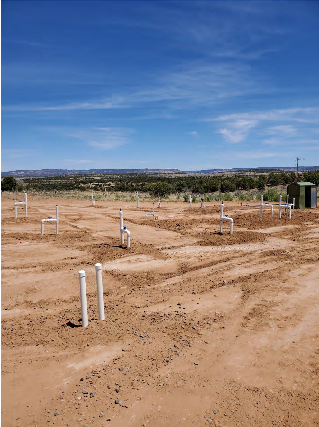
Photo 6: SVE installation complete.
