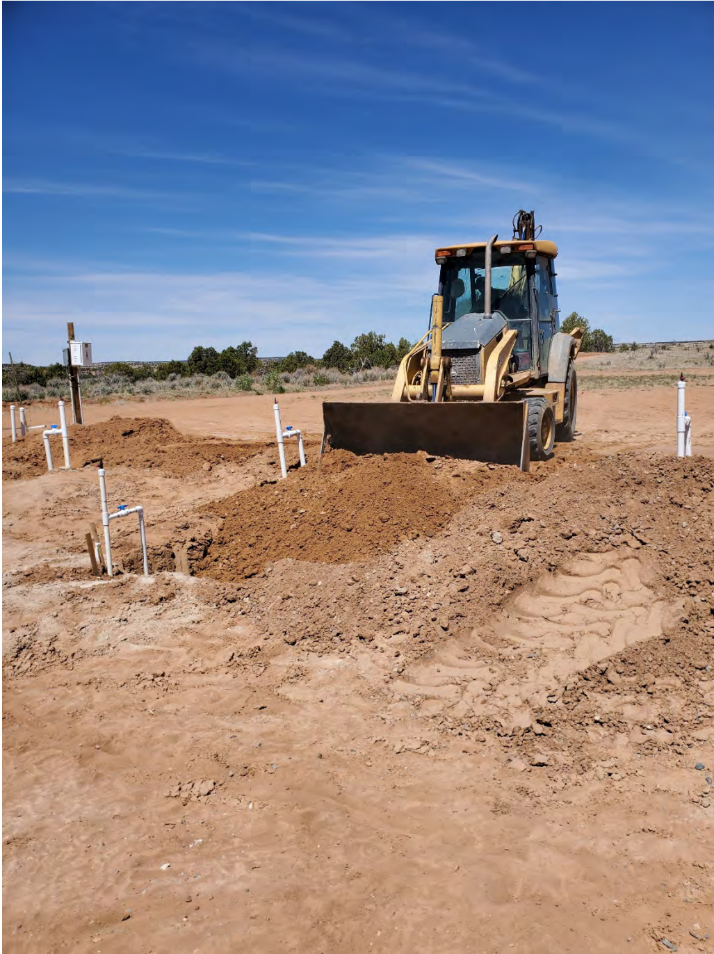
Photo 5: Backfilling trenches.
